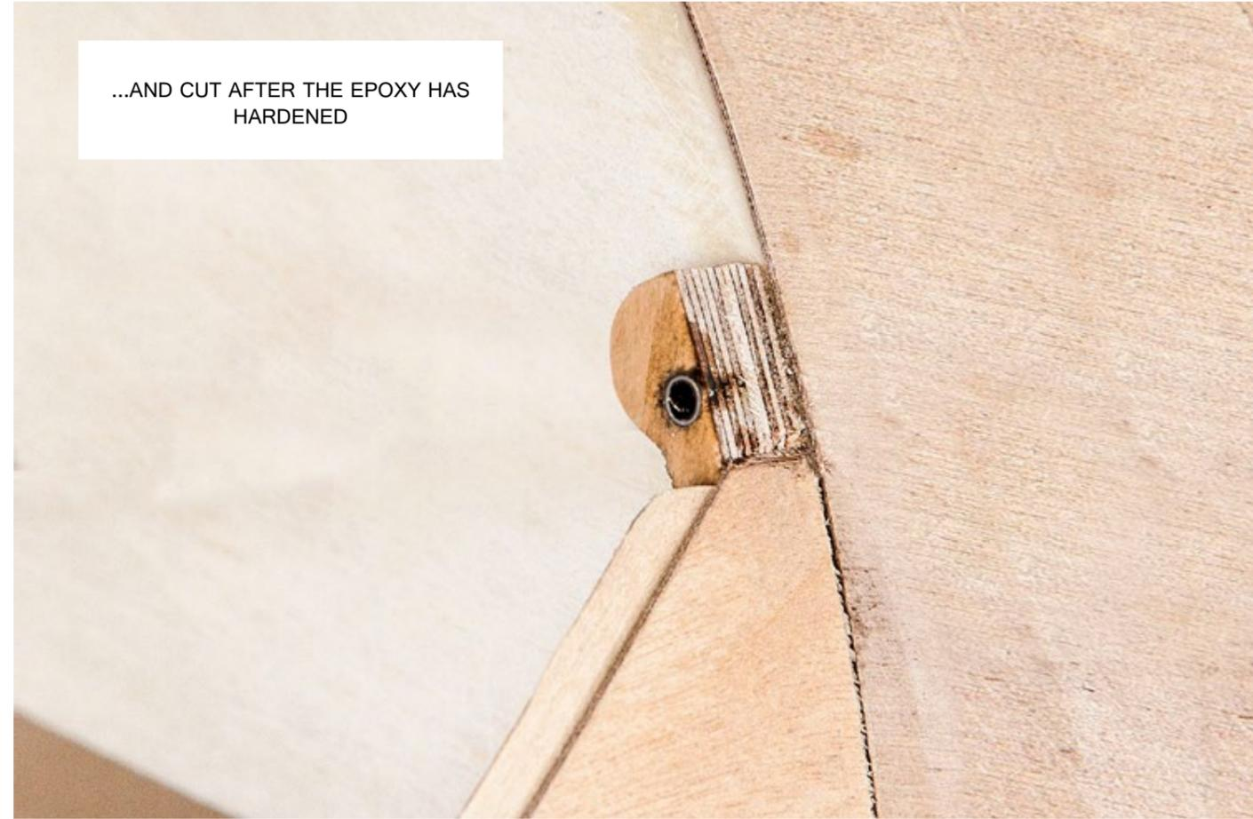
DRILL Ø 3 MM, GLUE THE TUBE WITH
